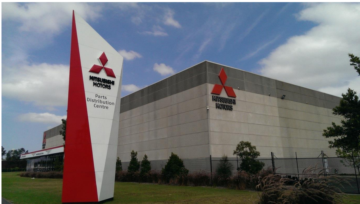
Figure: Mitsubishi Parts Distribution Centre in Clyde
