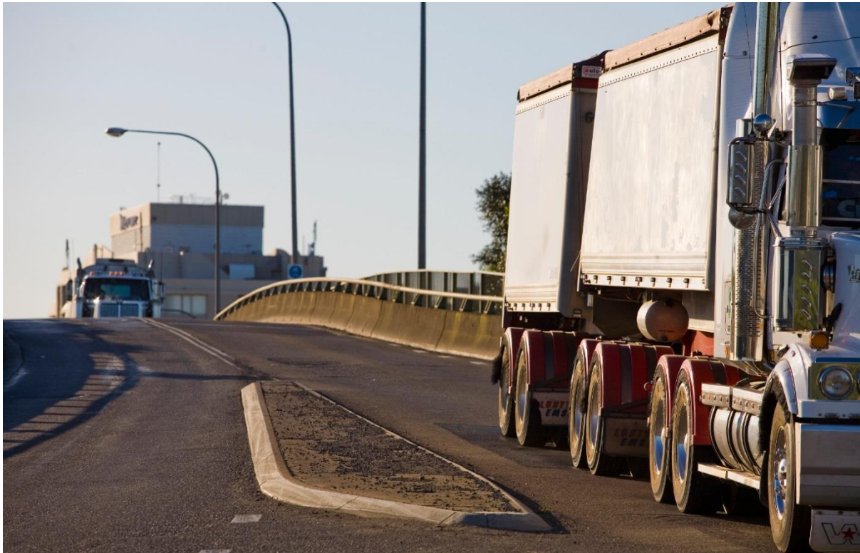
Figure: Grand Avenue Bridge – the main entry point into Camellia/Rosehill
