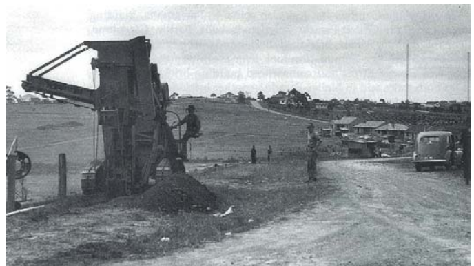
Preparing buildings sites and roads in Rydalmere for the Housing Commission c1945
